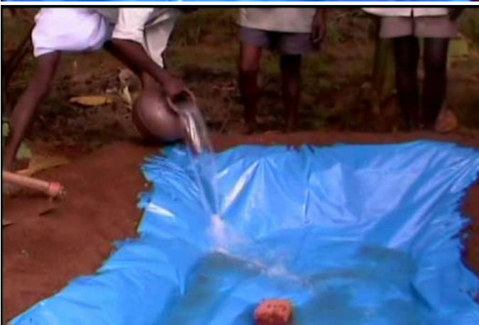
Now fill the pit with water. The depth of the water should be the same as the height of a brick. The water level must be maintained daily – if it goes down add more water. Even small holes in the sheet will result in water leakage.
