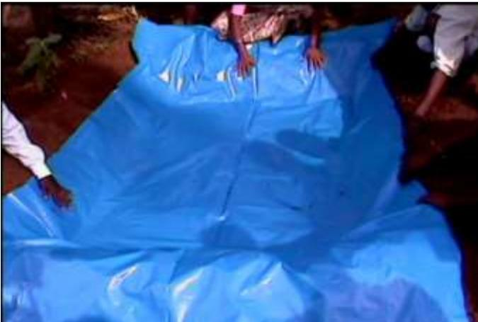
Spread out the plastic sheet. It should be 2 feet longer and 2 feet wider than the pit, with no holes. The sheet must be spread out smooth. The sheet's outer edges should be fixed with mud so that they don't move. Making this mud wall around the pit also helps to keep things out of the pit. Any mud that has fallen in should be removed completely.
